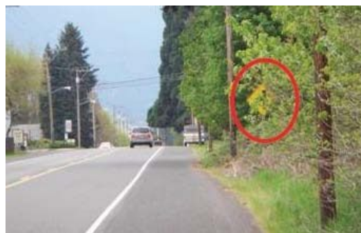
Figure 6. Hidden Road Sign that endangered all traffic users, including cyclists. (source : safety.fhwa.dot.gov)
